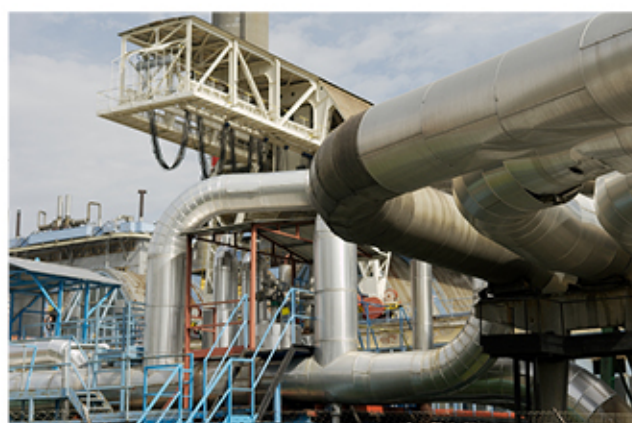
Heating facilities of various tanks
