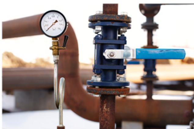
Pipe, water meter
