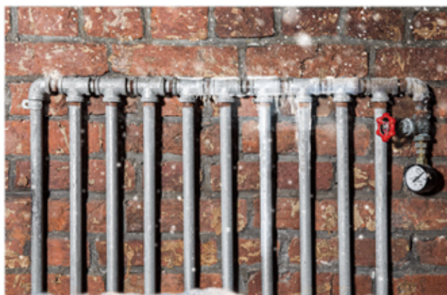
Various external piping
